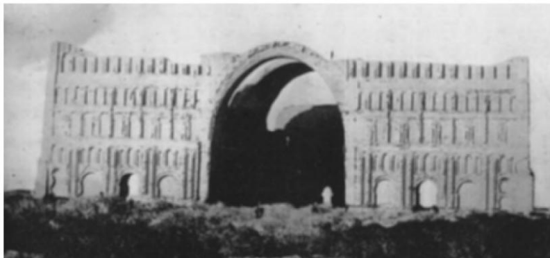
The Sasanians, rulers of Iran and adjacent areas in the centuries before Islam, maintained their capital at Ctesiphon, near present-day Baghdad. The main room of their palace was a giant iwān, a barrel-vaulted space, under which the ruler sat.
